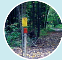
Pipeline markers do not indicate the exact location of the pipe.
