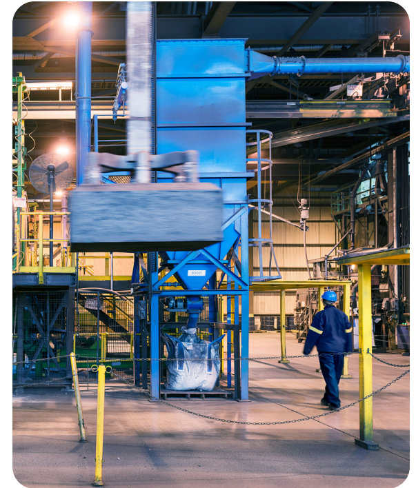
Industrial customer – aluminium sector
